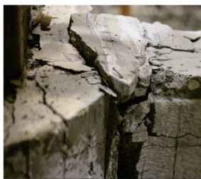
(e) SLJ 梁端 (e) Lintel-end of SLJ
