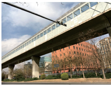
(a) 桥梁现场 (a) Bridge on-site
