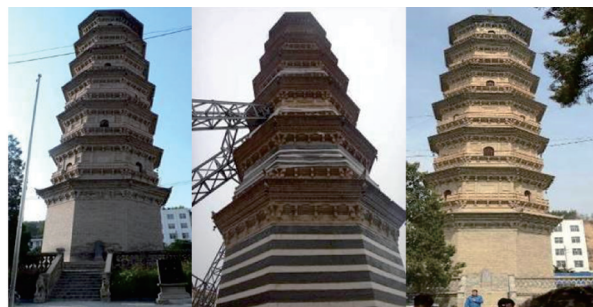
(a) 纠偏前 (b) 纠偏中 (c) 纠偏后 (a) Before deviation (b) Deviation rectification construction (c) After deviation rectification
