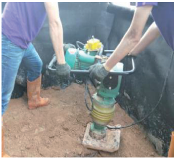
图 7 土体夯实 Fig.7 Soil compaction
