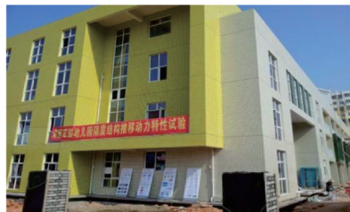
图3 建筑西南向立面 Fig. 3 Southwest elevation of building
